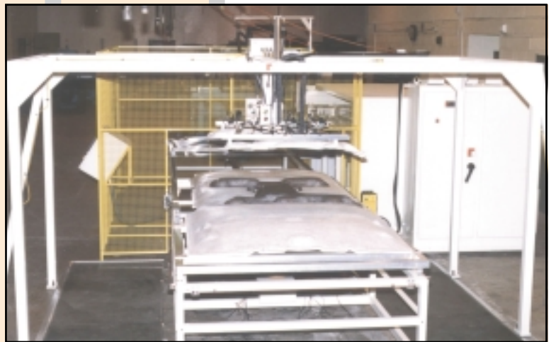
The vacuum pick-and-place mechanism raised after placing the air cap and lamp retainers on the dispensed headliner.
